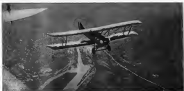
Type S-6 at 100 ft. above the factory at Middletown, N. Y.
